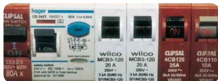
Image: Example of a switchboard with recommended safety devices
